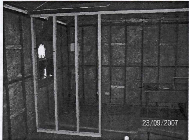
Work commences and framing for lining the hut.
