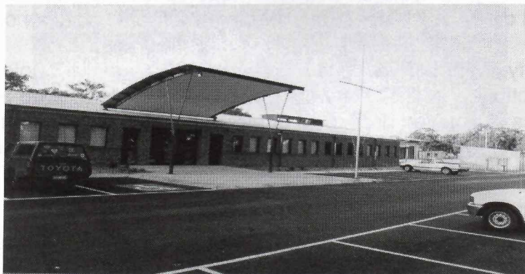
The new Passchendaele Barracks, Bendigo
